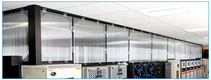
For airflow containment at the aisle level, the flexibility and onsite customization features of CPI's Build To Spec Kit (BTS) Hot Aisle Containment (HAC) contains the hot exhaust generated by existing, multi-vendor cabinets.
