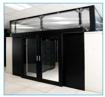
Sliding aisle containment doors seal the ends of the aisles without adding any additional clearance requirements. This solution integrates with perimeter cooling, provides immediate improved cooling efficiency and is compatible with economization methods.
