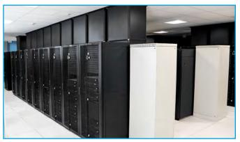
The cabinet solution includes CPI's GF-Series GlobalFrame® Gen 2 Cabinet with Vertical Exhaust Duct, Monitored eConnect® PDUs and cable management accessories.
