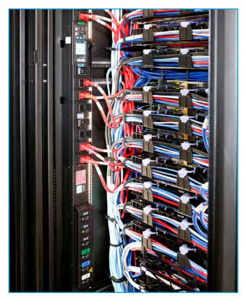
CPI's Monitored eConnect<sup>®</sup> PDUs support two temperature and humidity probes providing temperature and humidity measurement at each cabinet, and feature Secure Array<sup>®</sup> IP Consolidation technology, which greatly reduces the number of networking ports required for the PDUs.
