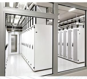
and the addition of collars on air handler units in order to create a complete closed return, and ducts to be placed above each cabinet. The ducts must be able to extend to the overhead plenum
